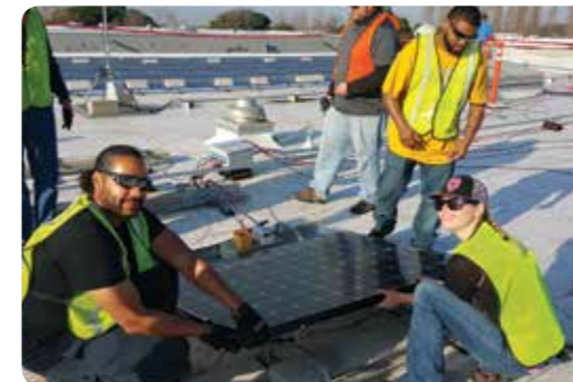
Teamwork to take this roof solar
